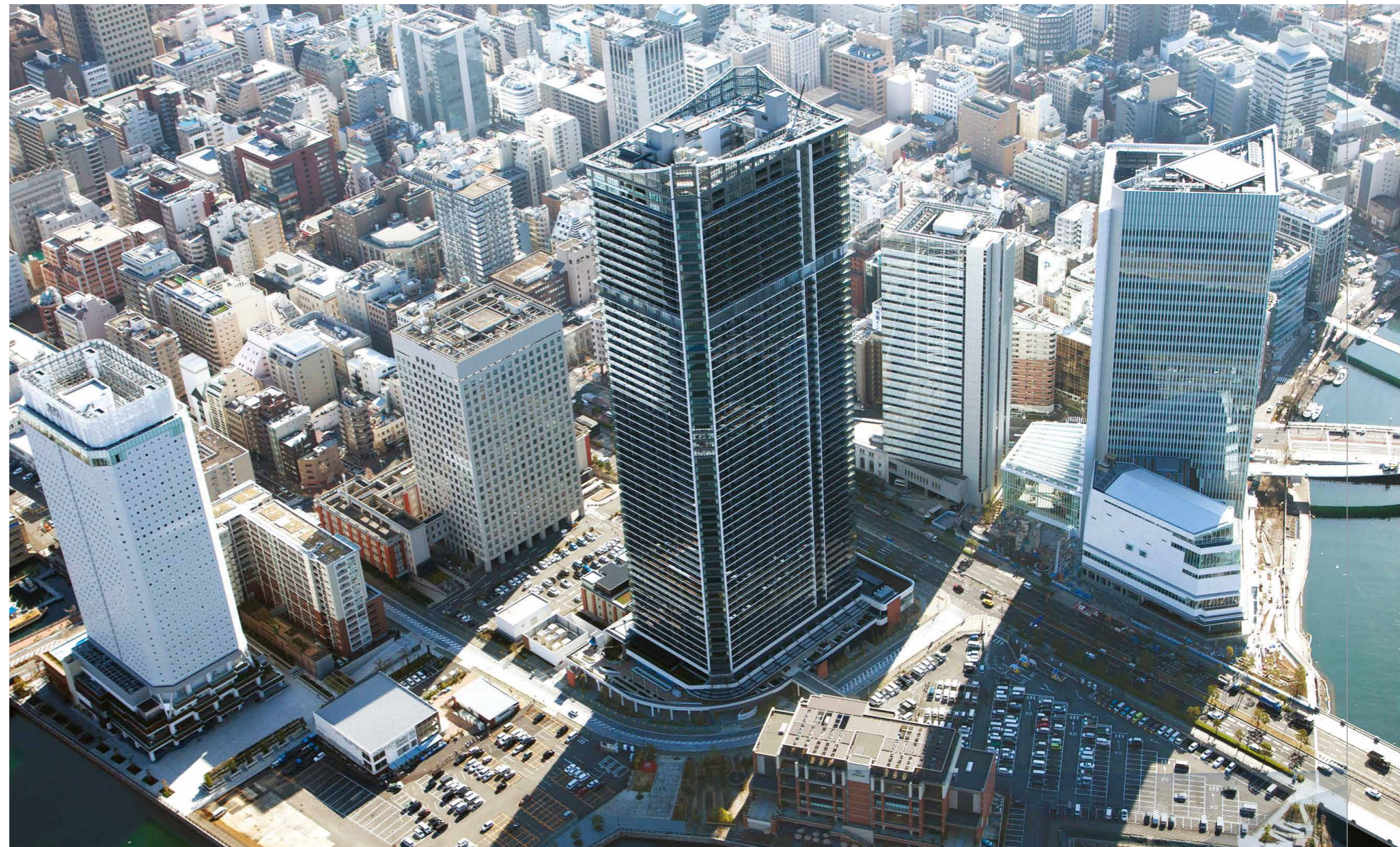
Oakwood Suites Yokohama occupies the 46 th to 51 st floors of The Kitamaka Yokohama Tower, Yokohama's tallest and largest residential complex.
