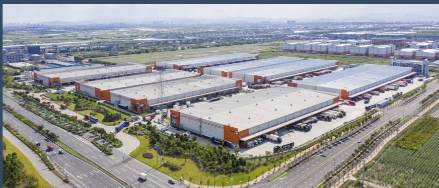
▲ Mapletree (Yuyao) Industrial Park Phase I and Phase II consist of eight single-storey warehouses, strategically located between Ningbo and Hangzhou, two major cities in the Yangtze River Delta, and connected to multiple highways.
