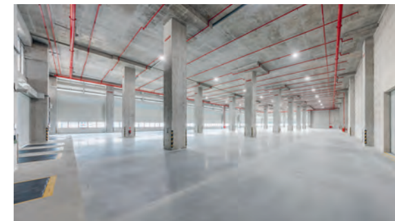
Above: Interior features such as high clear heights, strong floor loading and superflat flooring support automation and optimise storage efficiency.
