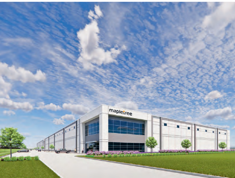
Above: Mapletree recently broke ground on a 312,306-square-foot industrial warehouse at 3600 Houbolt Road in Joliet, Illinois.
