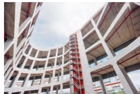
Below: Ramp design enables direct vehicular access to all warehouse units.
