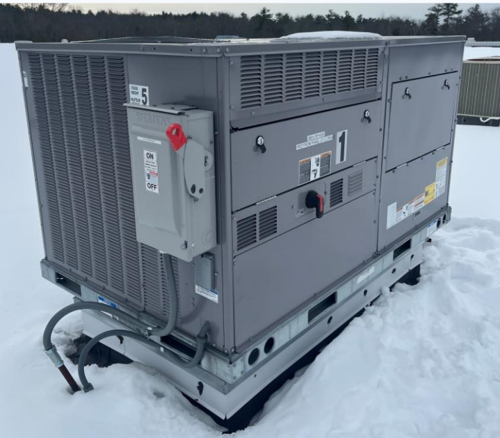
New electric heat pump rooftop unit
