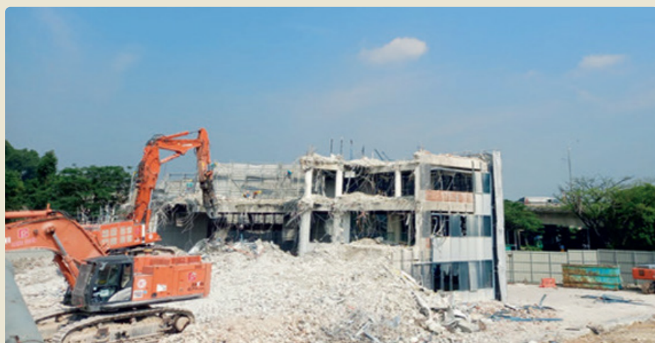
98% of construction materials were recycled during the demolition at Mapletree Joo Koon Logistics Hub in Singapore
