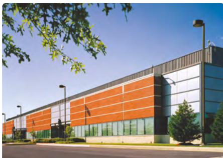
Acquired in 2019, 44490 Chilum Place, Ashburn is a fully fitted hyperscale data centre located in Virginia, US.
