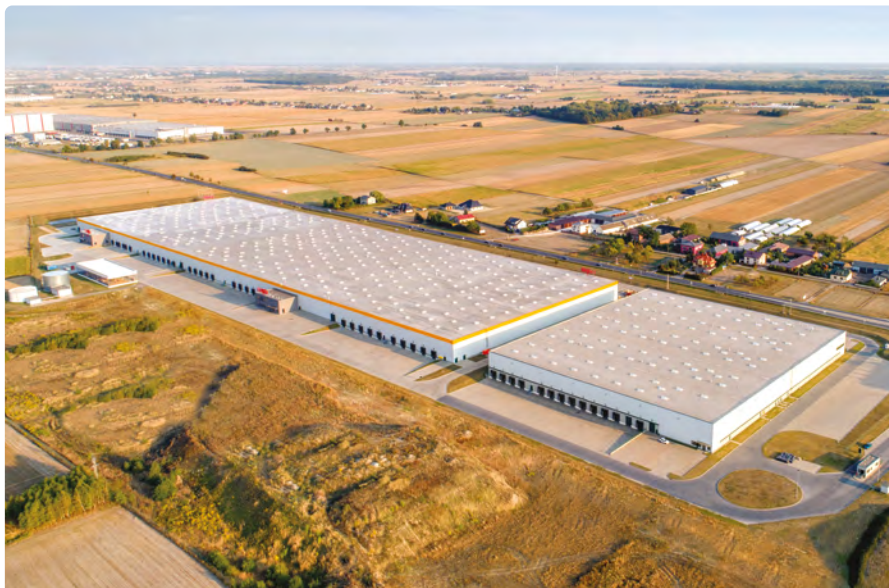
Mapletree secured the largest warehouse lease in Poland in 2025, which comprised 128,000 sqm of space across Piotrkow II DC1, Piotrkow II DC2 and Piotrkow II DC3.
