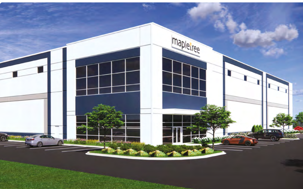
When complete, 1360 Schiferl Road in Bartlett, Illinois, will feature 36-foot clear heights, 42 dock doors, two drive-in doors and 181 car parking spaces.
