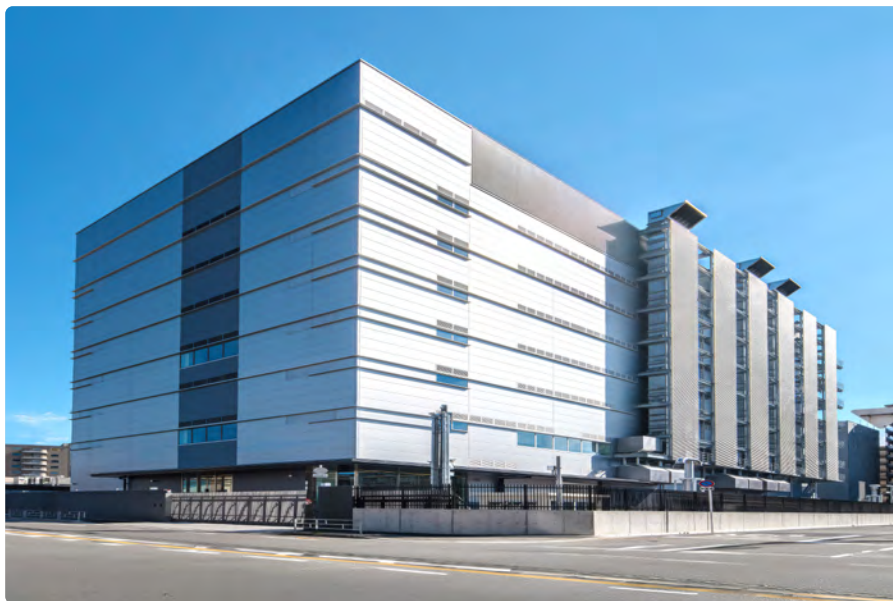
In May 2025, MIT completed the final phase of fitting-out works at Osaka Data Centre in Osaka, Japan.
