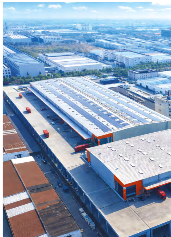
In FY25/26, Mapletree (Suzhou) Modern Service Intelligent Park achieved LEED Zero Energy certification.
