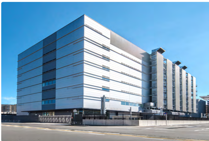
In May 2025, MIT completed the final phase of fitting-out works at Osaka Data Centre in Osaka, Japan.
