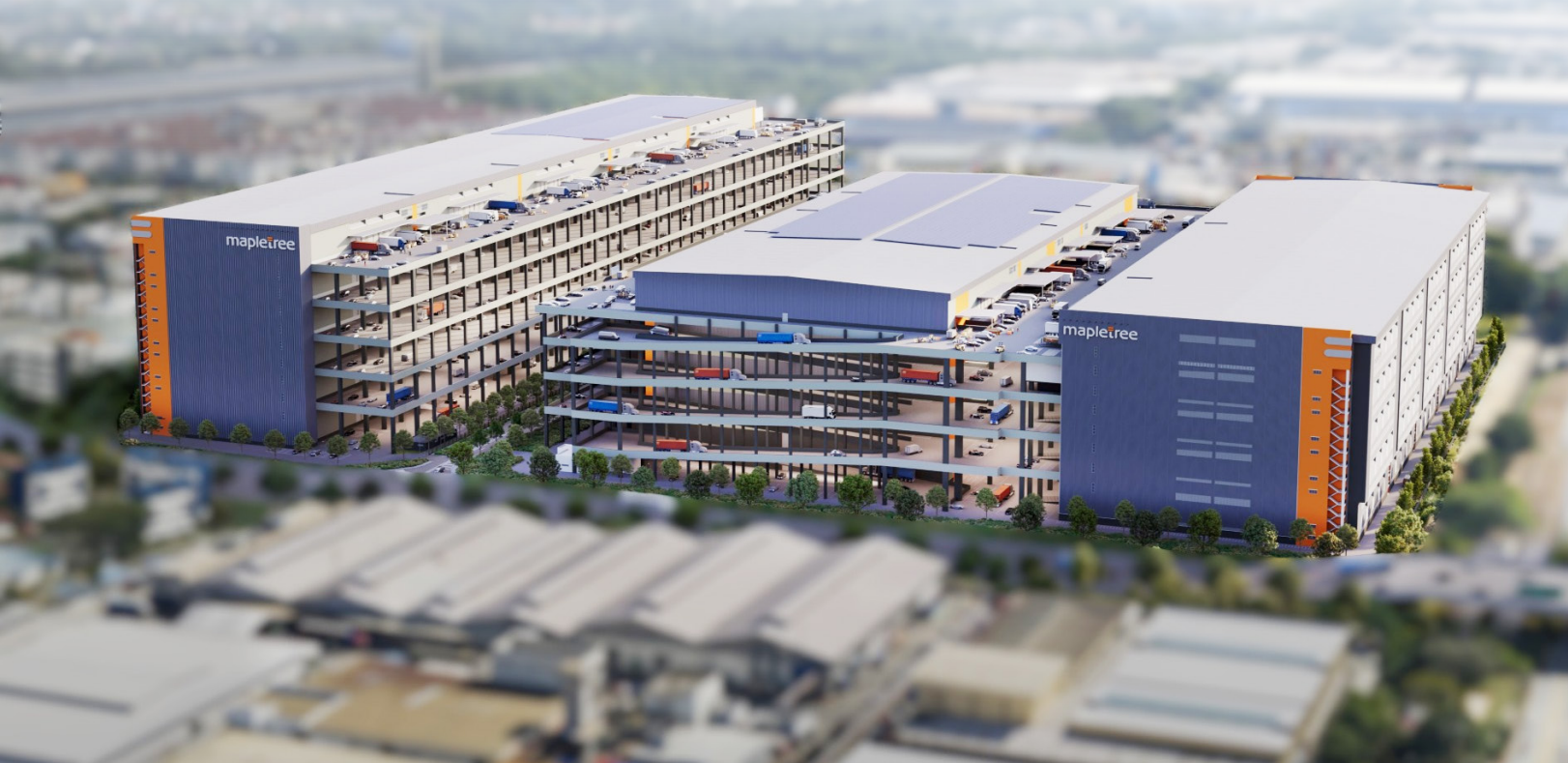
▲ With a net lettable area of 452,786 sq m, Mapletree Logistics Hub — Ulas Shah Alam is one of Malaysia’s premier logistics developments and a project under the MEGA fund.
