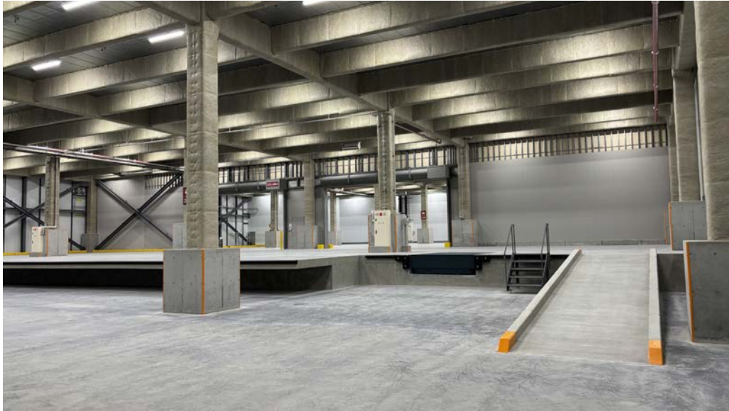
▲ Chitose Kami-Osatsu Logistics Centre is a modern three-storey facility that is well-positioned to meet rising logistics demand in the area.
