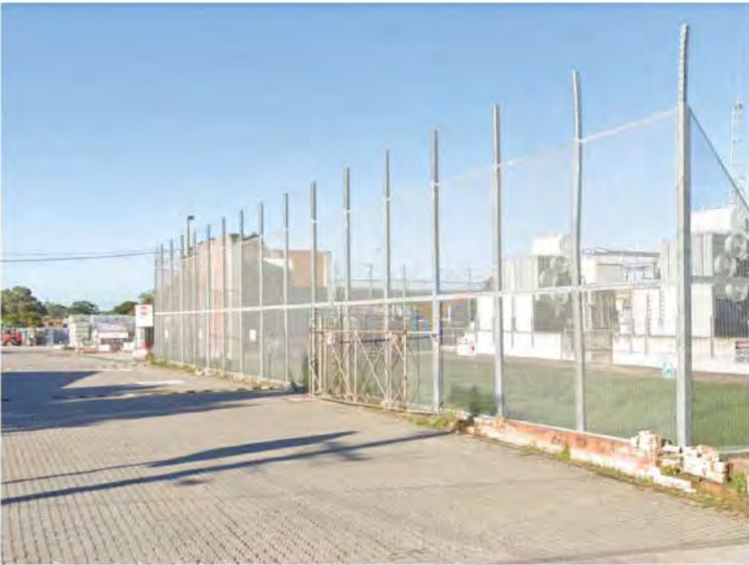
IMAGE - FENCE TYPE 3 - EXISTING AT 24 KELSO CR SUBSTATION
