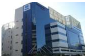
Light Industrial Buildings
