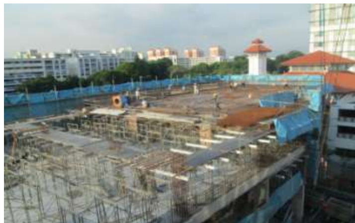
▲ Formwork and rebar installation
