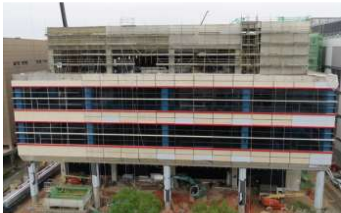
▲ Construction works in progress
